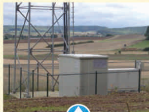
Lightweight cabinets and shelters for mobile communication sites, simplifying transportation to remote or difficult locations, such as by helicopter to building rooftop installations.
